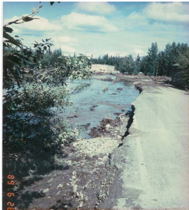
Photo 3: Central erosion from Crooked Creek at mile 128 past the Steese Highway bridge, with DOT/PF shop in the background, 1989.
